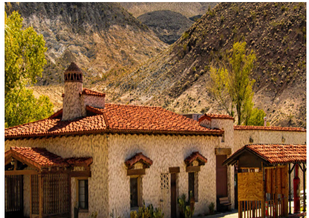
Former garage converted into the Visitor Center destroyed in the 2021 fire
