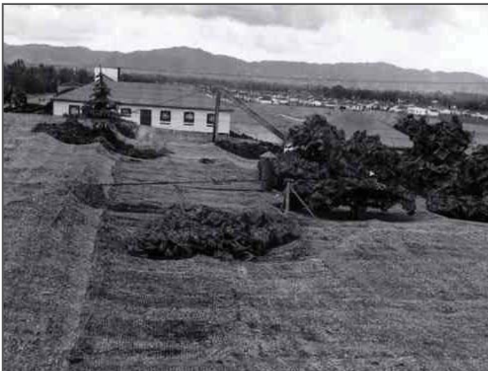
Fake trees and shrubs made from chicken wire were treated with adhesive, then covered with chicken feathers as leaves and painted various shades of green and brown.
